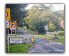
The village gateway helps to create 'a sense of place' when drivers enter the village, and the physical measures are designed such that drivers are required to slow down before entry.
