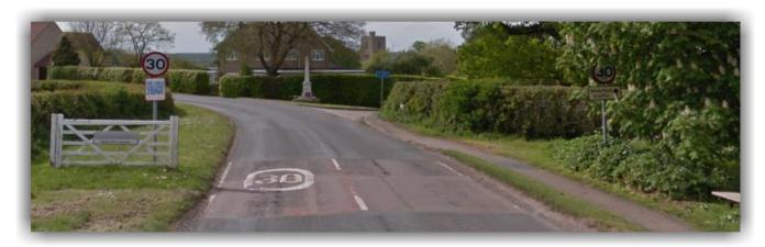
These gateways only have signs and lines, and always display the village name to introduce drivers to the village. In addition, road markings are used to create a visual impact when drivers enter the village. These markings could be:
