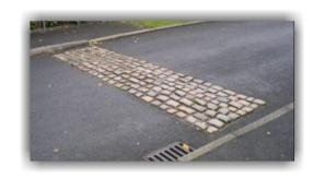
Rumble devices are small, raised areas across the carriageway with a vibratory, audible and visual effect. They are used, usually in rural areas, to alert drivers to take greater care in advance of a hazard such as a bend or junction. In combination with a gateway, they can indicate the entry to a village or the start of a series of traffic calming measures. They have also been used to designate the start of shared use roads in new developments.
